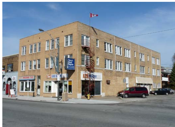
Figure 68. Leatherdale Block located at 1380-1394 Wyandotte Street East
