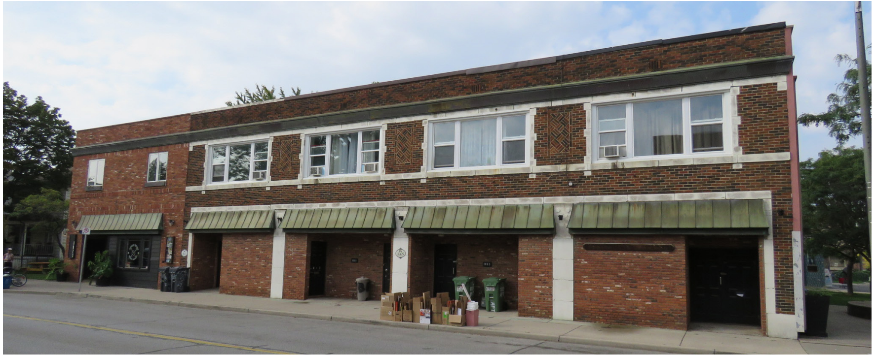
Figure 100. A building facade on the west side of Drouillard Road with original storefront windows and doors bricked in, eliminating the connection with the street
