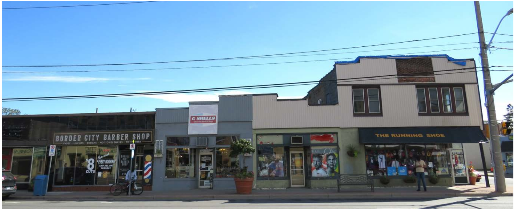
Figure 113. Building facades along the south side of Wyandotte Street East in the Pillette Village BIA, where aluminum siding covering the original brick
