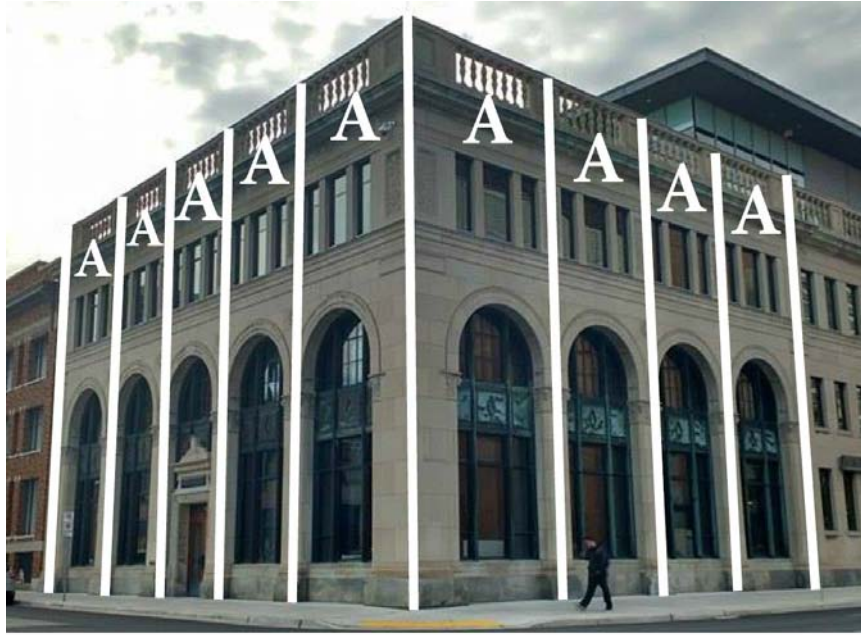
Figure 31. Former Windsor Star building showing a repeated “A” rhythm pattern
