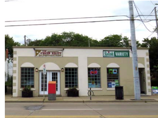
Figure 127. Windows are barred over and cluttered with merchandise and signage. Non-traditional cladding is used on the facade.
