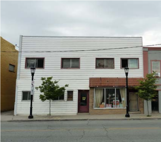
Figure 55. 3236 Sandwich Street before renovations
