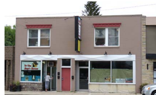
Figure 131. Original brick has been painted over, and non-traditional building materials have been added on top
