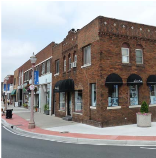
Figure 20. Erie Street and Parent Avenue, Windsor
