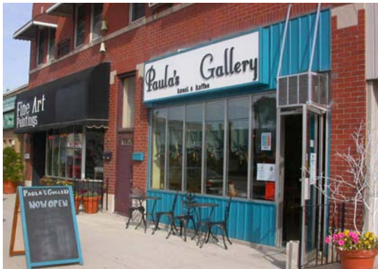
Figure 21. Wyandotte Street E, Windsor
