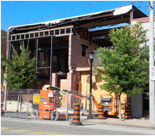
Figure 56. 3236 Sandwich Street during renovations
