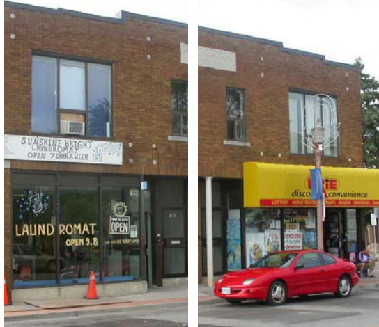
Figure 36. Window on the left is open whereas on the right it is blocked with signs
