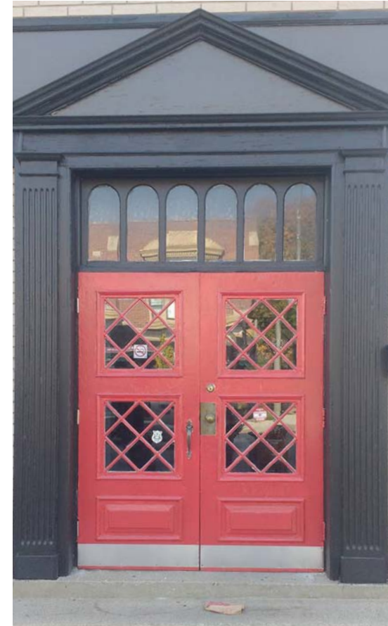
Figure 54. Distinct doors can make a business more visible and improve the overall appearance of the storefront
