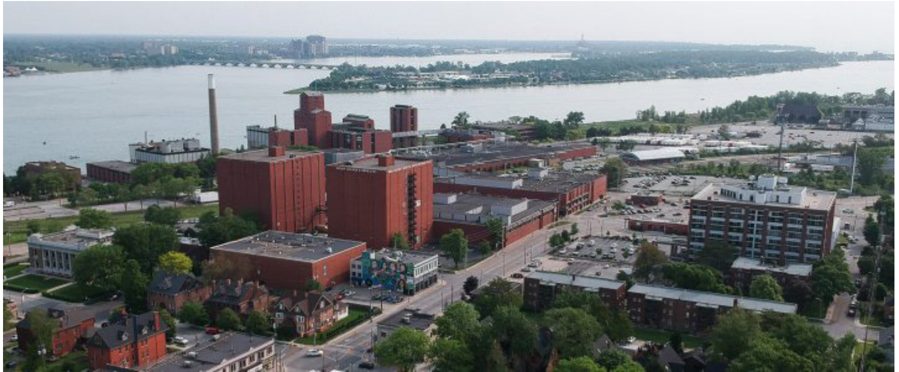
Figure 2. Overhead view of the Walkerville St. E. Main Street in the Walkerville BIA.
