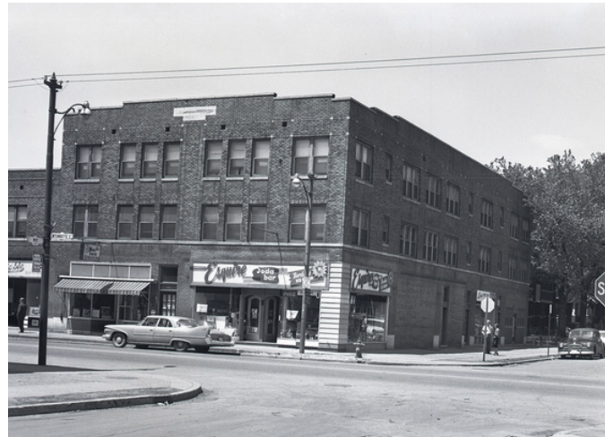
Figure 67. Leatherdale Block located at 1380-1394 Wyandotte Street East (1960)
