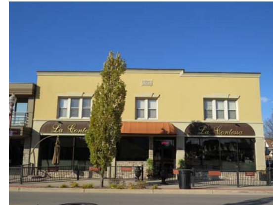
Figure 139. This traditional Main Street building has been covered with non-traditional materials
