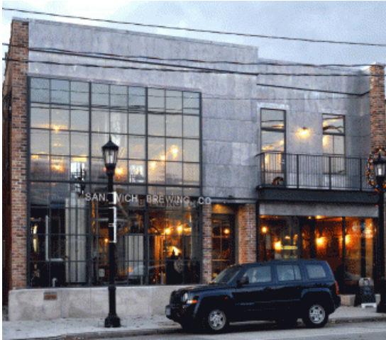
Figure 57. 3236 Sandwich Street at completion
