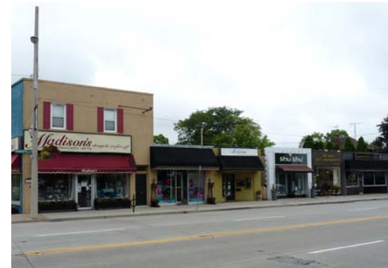
Figure 39. A continuous street wall is desirable such as this example along Wyandotte Street East in Olde Riverside
