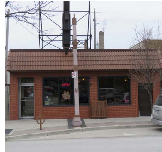
Figure 50. The store front in Figure 49 is enhanced by constructing open glass windows making the storefront more inviting to the public by creating a visual connection with the public realm.
