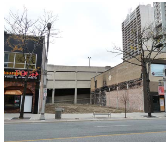
Figure 40. Avoid large breaks in the street wall such as this example along Ouellette Avenue
